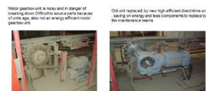
Projects – Setting motor and gearbox
